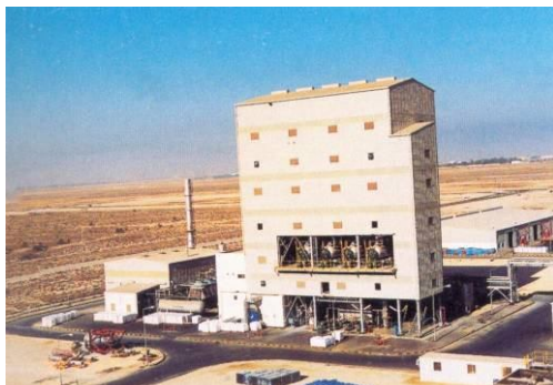
GRANULAR PARAFORMALDEHYDE PLANT
